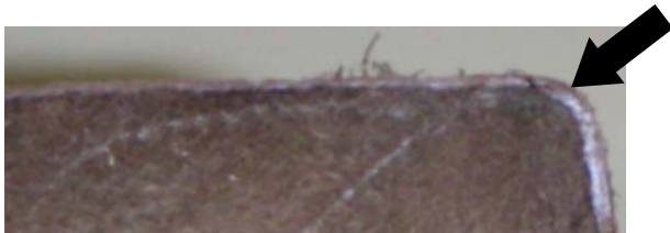
The Horizon decking surface is not compromised.
