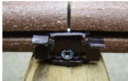
B. End Seam Fastener Application
