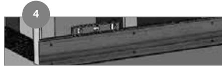
Secure the end of the board using two #8 x 2 1/2 in. composite decking screws, not closer than 1 1/2 in. from the board end and 1 in. from the board edge. Pre-drill end fasteners to prevent stress cracking.
