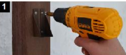
1 Attach Brackets : Use chart to find rail heights. Measure up from ground, mark post for bracket bottom. Attach with provided screws. Secure rails into brackets with screws.
